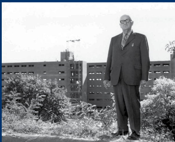
Frank Campbell during construction of Campbell Hall (1972)
