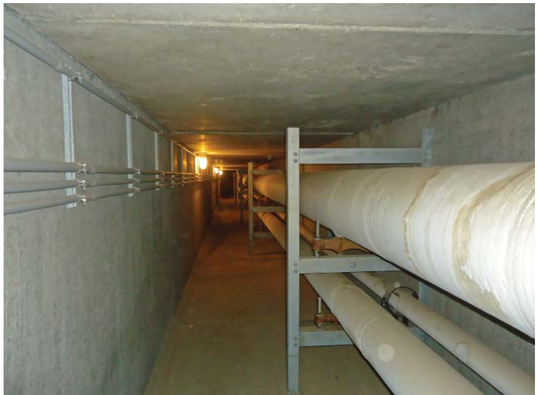
Graphic 3.25 Underground Steam Tunnel Clarion Campus
