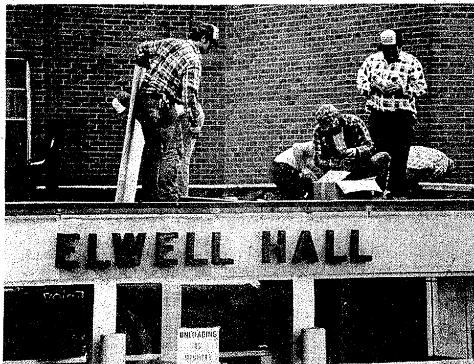
Workers make noise and progress as Elwell's leaky roofs are finally fixed. (Photo by Bob Finch)
