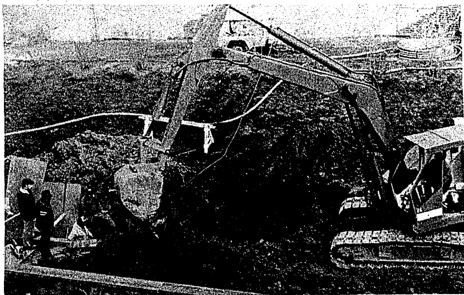
Workman repair the water main break outside Montour Hall.
