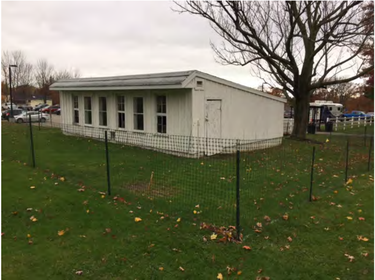
Figure 5 - Overview of the Chicken Coop with fence installed
