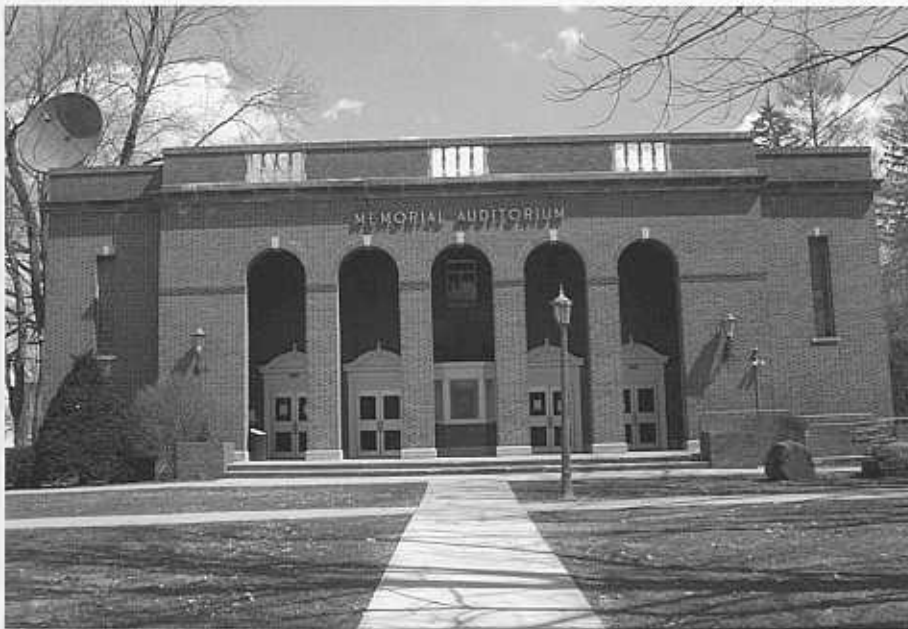
The renovation of Memorial Auditorium was authorized by the Pennsylvania Legislature. While original bids came in over budget, the project is currently being redesigned with a tentative rebid date of November 2001 with completion anticipated in July 2003.
