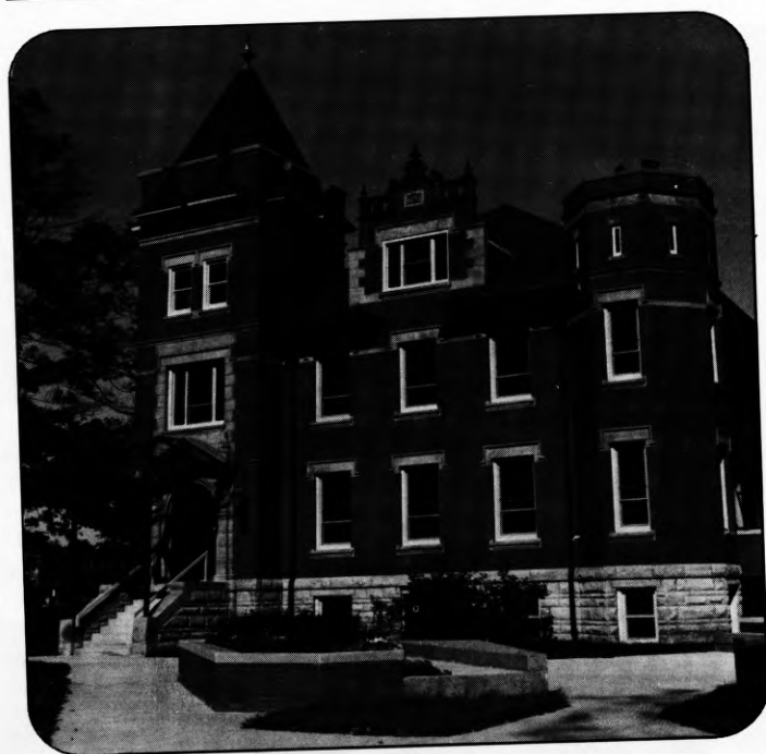
Center for the Performing Arts
