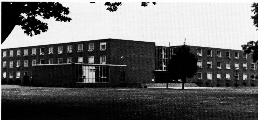
Centennial Hall – Women's Dormitory
