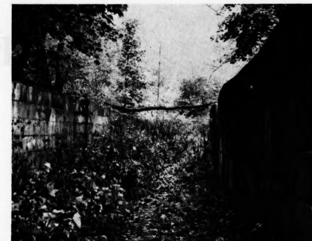
Part of the "Old Lock" in Sharpsville.
