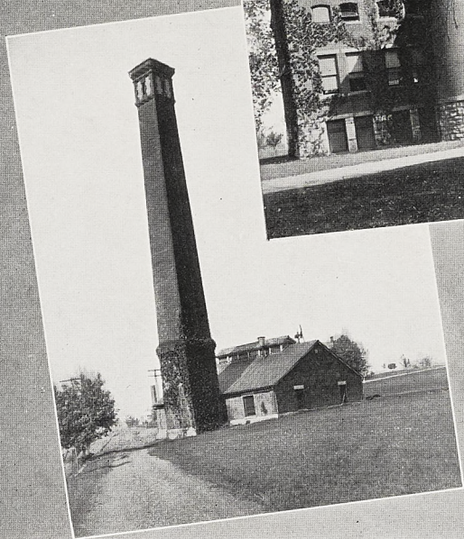
THE HEATING PLANT
