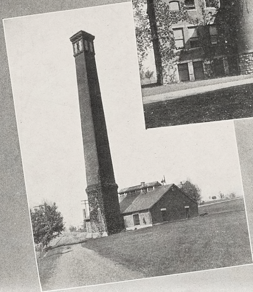
THE HEATING PLANT
