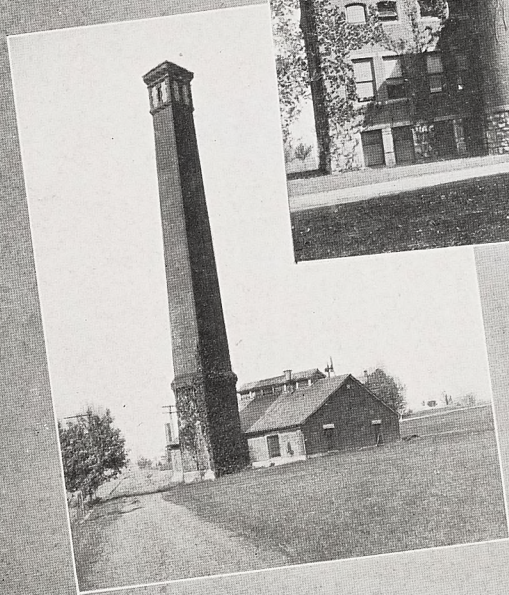
THE HEATING PLANT
