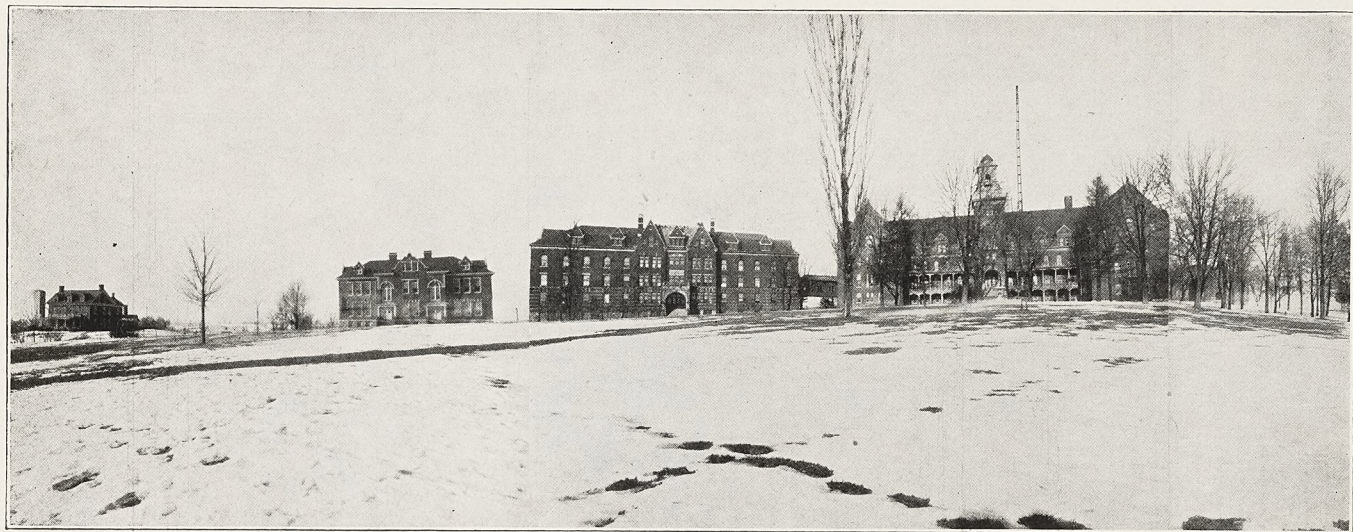
BUILDINGS AND GROUNDS
