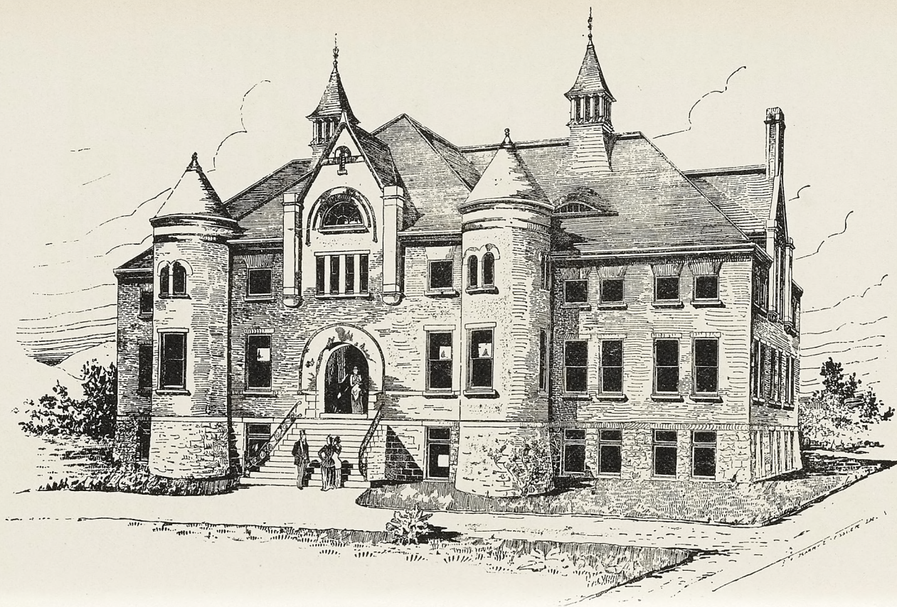
NEW GYMNASIUM BUILDING.
