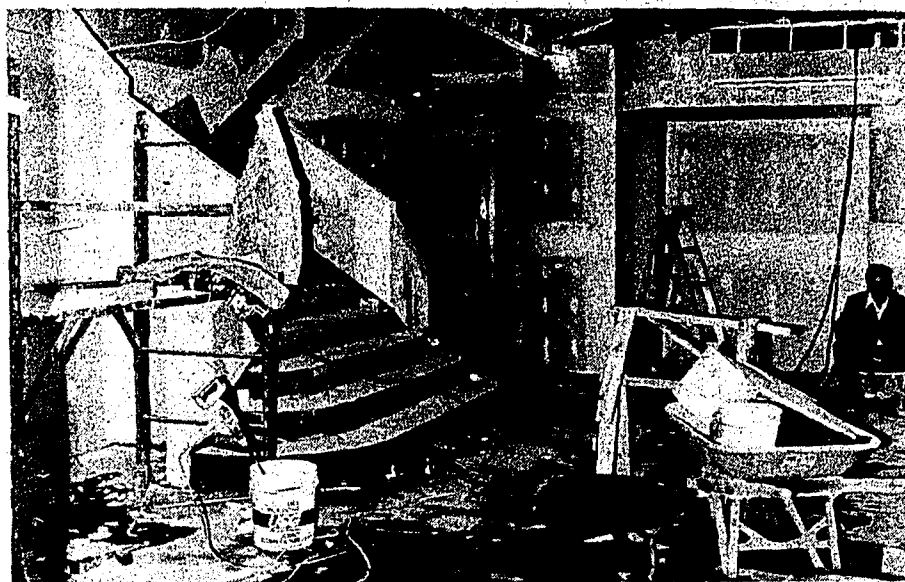
Renovations continue on the Columbia Theatre which is now the new home of the BTE.
