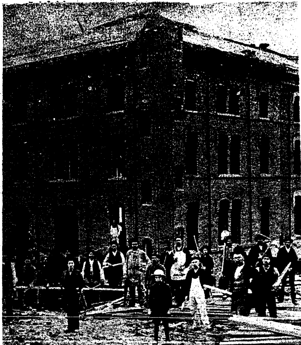
The construction crew which built the second of three sections of Waller dormitory, takes a break in the action to pose for a photographer. Wonder if their union officials had to bargain for time off? Circa 1890, compliments of the BSC Public Relations Office.
