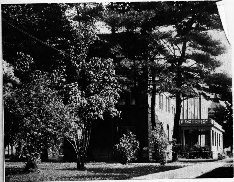
NORTH END OF HAVEN HALL, WITHOUT ADDITION
