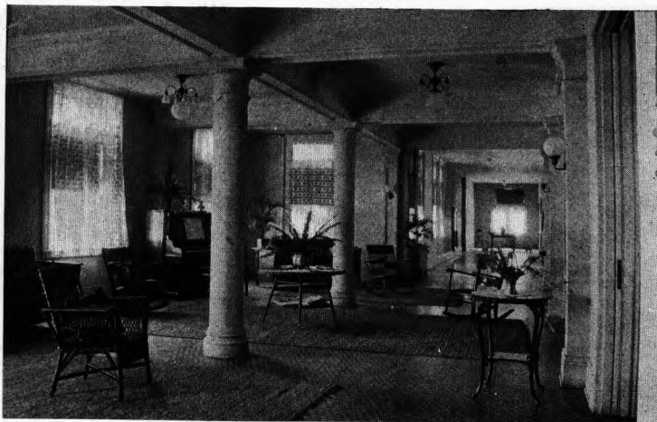
CORRIDOR OF HAVEN HALL
