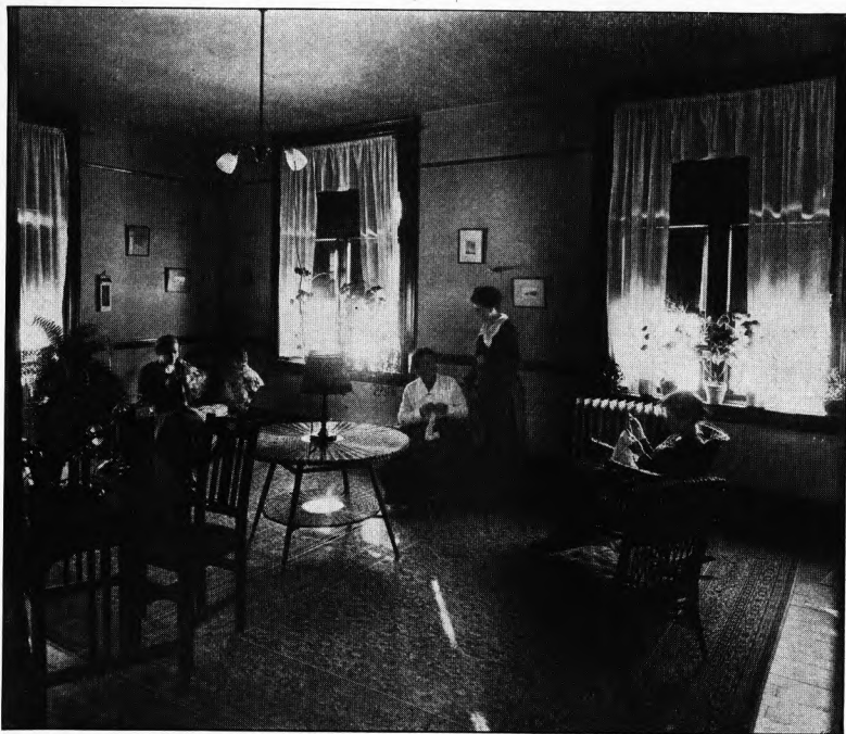
MATRON'S ROOM IN HAVEN HALL
