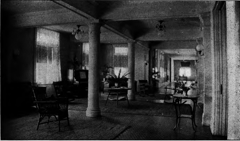
CORRIDOR OF HAVEN HALL
