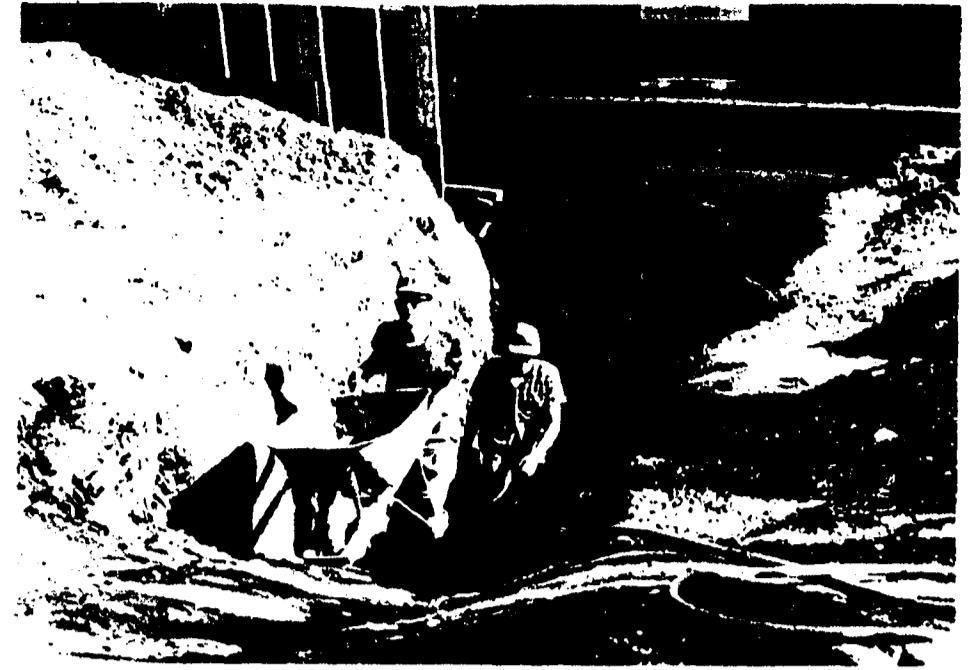
Workmen come back into the daylight after spending time in the underworld of the moleman. Construction of the new Adapted Physical Education Center is expected to be completed by January.
