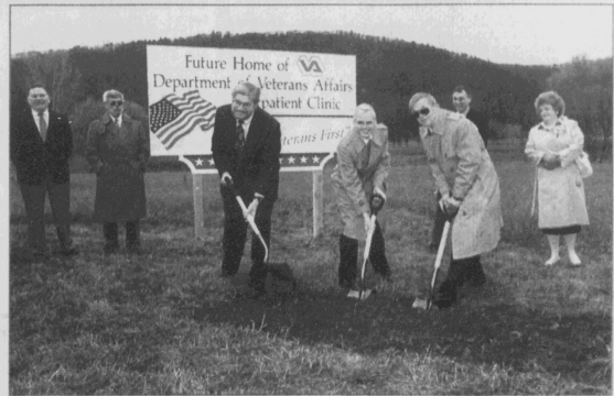
The first shovelfuls of dirt for the construction of the new Sayre Veterans Outpatient Clinic in Athens Township were ceremoniously dug by (left to right): Dr. Robert L. Jones, network director, VISN No. 4; Reedes Hurt, director of the Wilkes-Barre Veterans Administration Medical Clinic; and Dr. John Wilt, chief medical officer at the Sayre Outpatient Clinic for the Department of Veterans Affairs. (Review Photo by Bonnie West)
