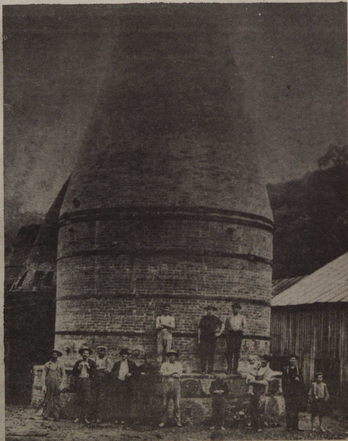
"Both coal and wood are used for fuel. Wood is used for finishing the burning, it is said, because it gives more blaze than coal, enabling the burner to finish the ware in better shape."
