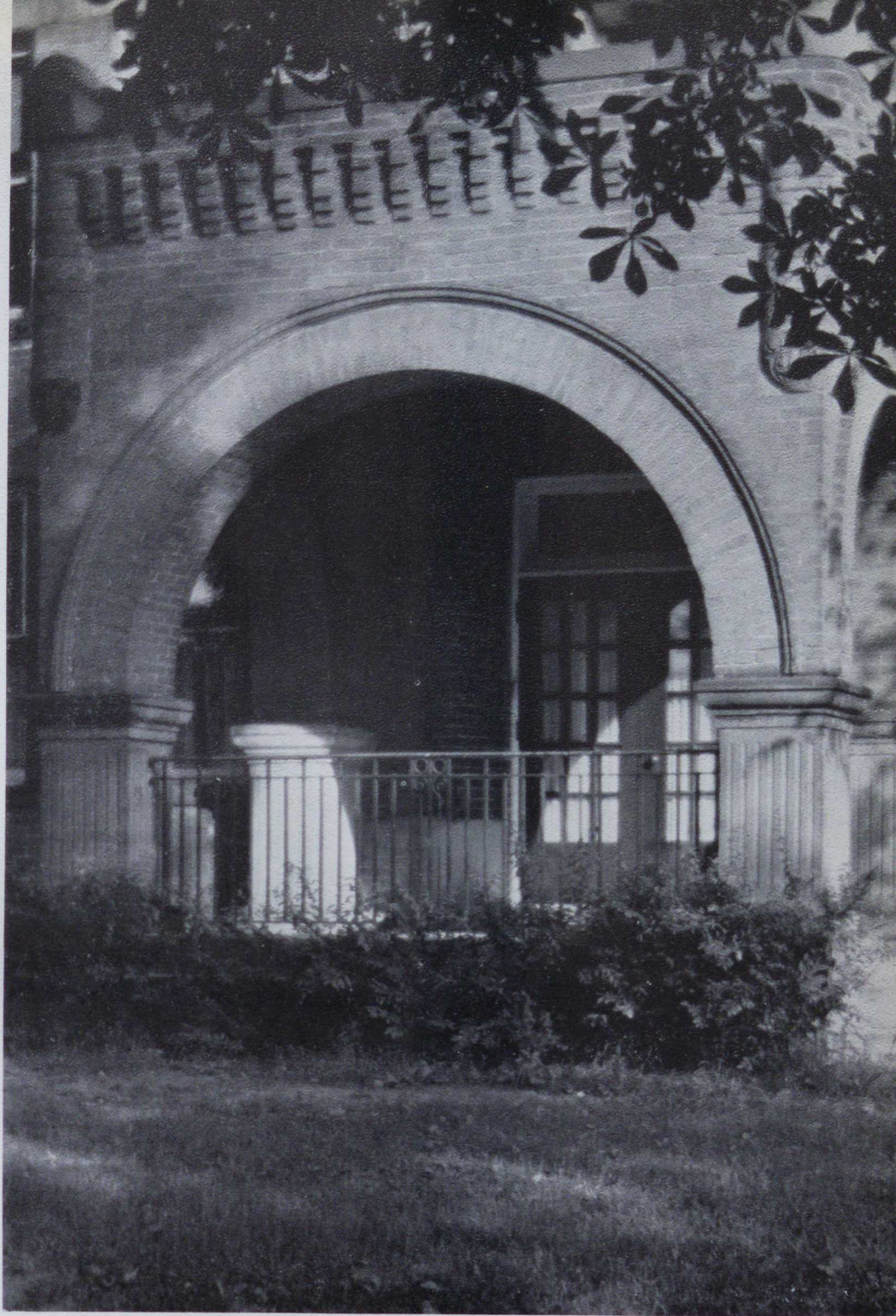
North Hall Entrance
