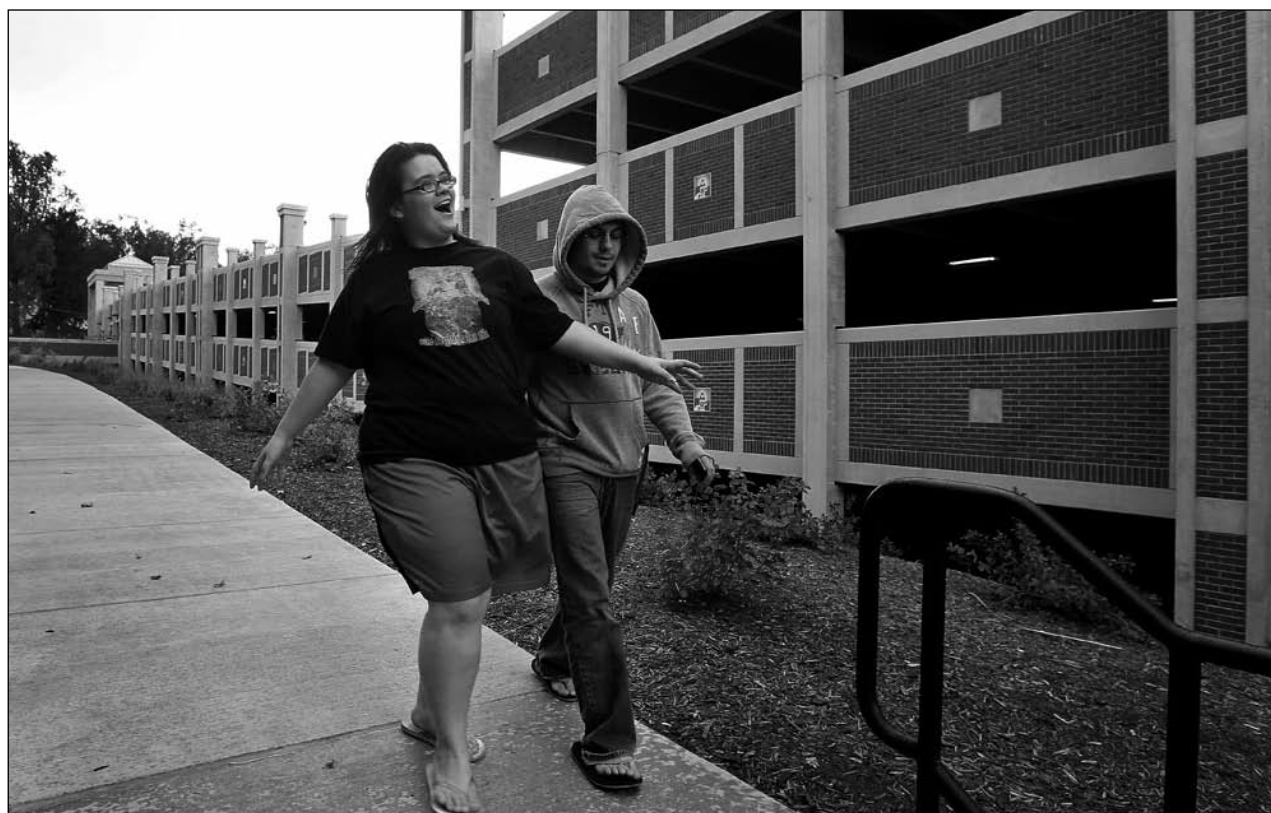
Vulcan Garage is a 660-space facility, with 375 spaces set aside for hourly parking. The garage is averaging 616 cars per day.
