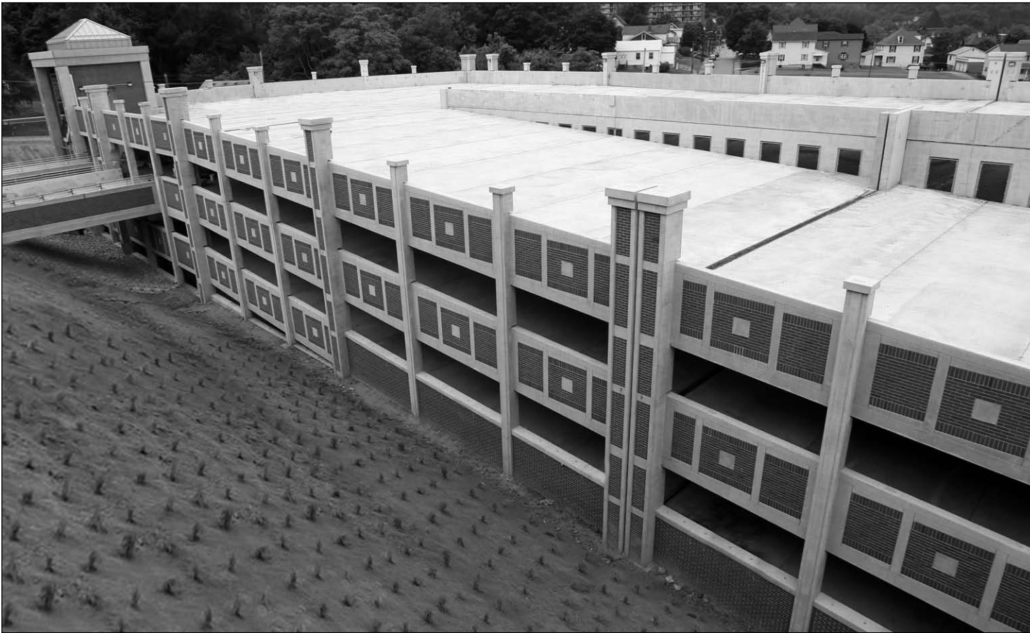
Coinciding with the start of the new academic year is the opening of the Vulcan Garage, a 661-space parking facility beside Manderino Library.
