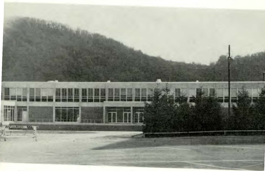
HAMER GYMNASIUM AND NATATORIUM
