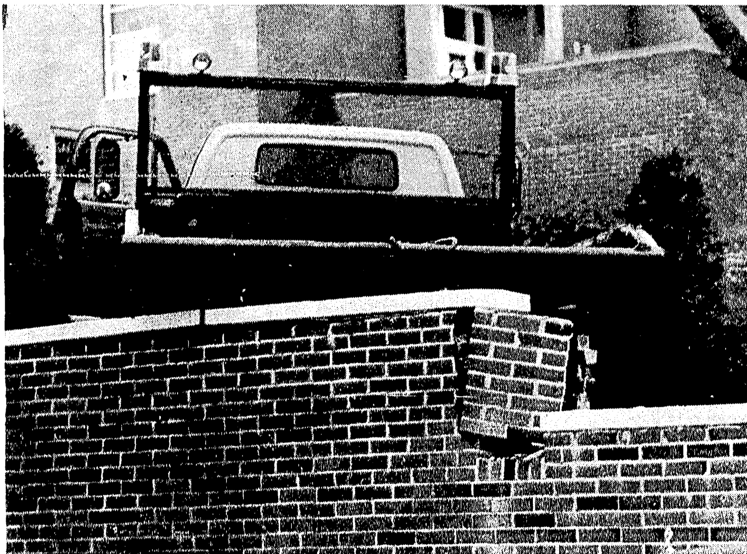
WHAT HAPPENED HERE? This incident occurred on Tuesday, at Lycoming Hall. Since the Security Department would not give the Campus Voice any information explaining this happening, information will be provided at a later date.
