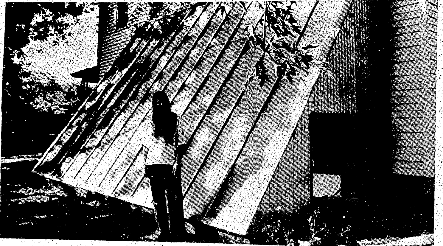
Rays are collected in a solar panel with water and are pumped through by a motor which is powered by a 12 volt battery.
