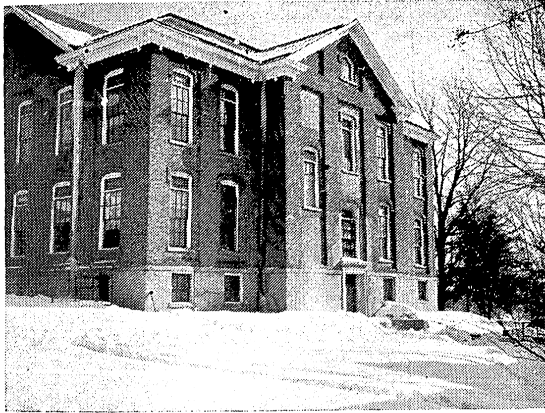
Pictured above is historic Noetling Hall, which will undergo extensive renovation commencing this summer.
