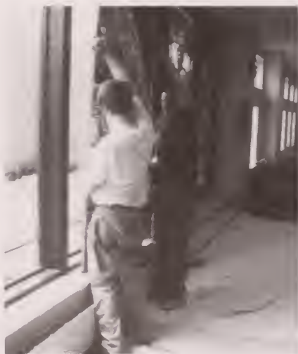
Peter Koch (foreground) and his assistant ease the Tiffany windows out of their place in the library so they can be clean and reinstalled farther from the window so air can circulate and keep the windows cool.
