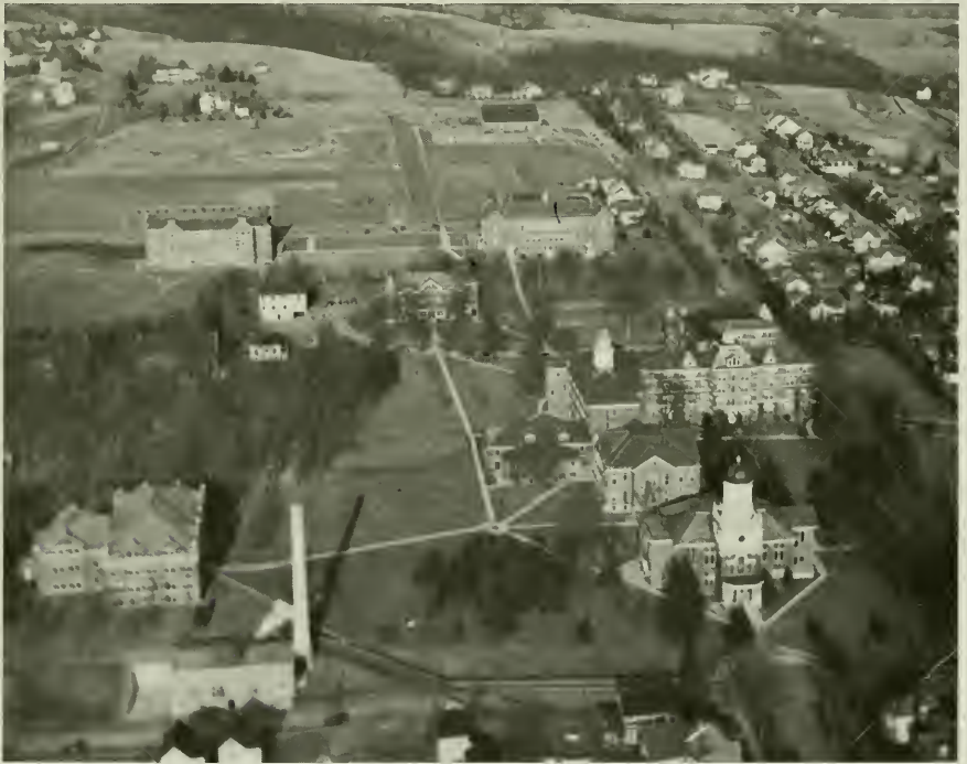
This aerial photograph, taken in the early 1940s, shows the campus as it remained until the massive building program began in the early 1960s.
