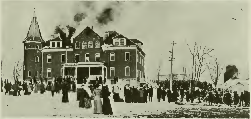
Fire in employees' dormitory on February 4, 1904. Building was named North Hall in 1908.
