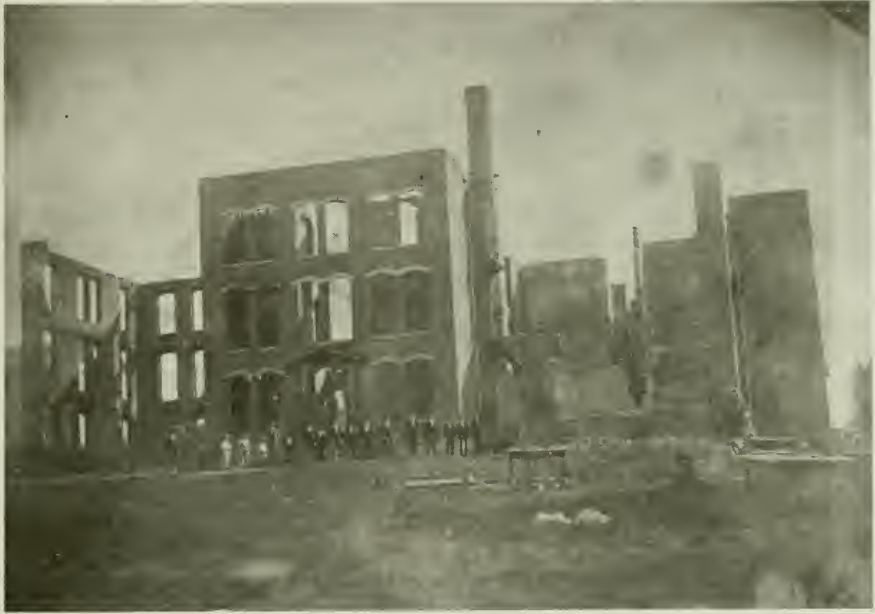
Remains of dormitory after fire of September 4, 1875.
