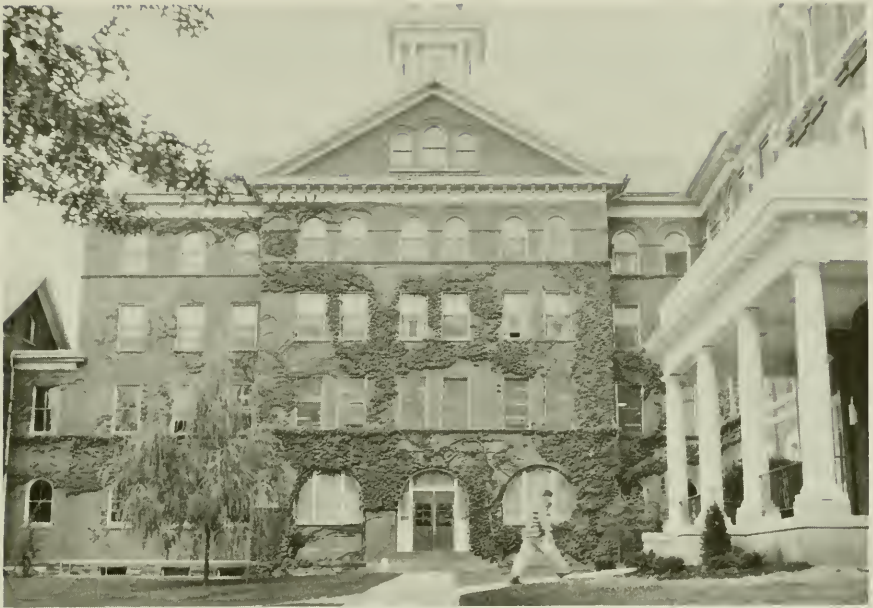
North wing of Waller Hall before demolition.
