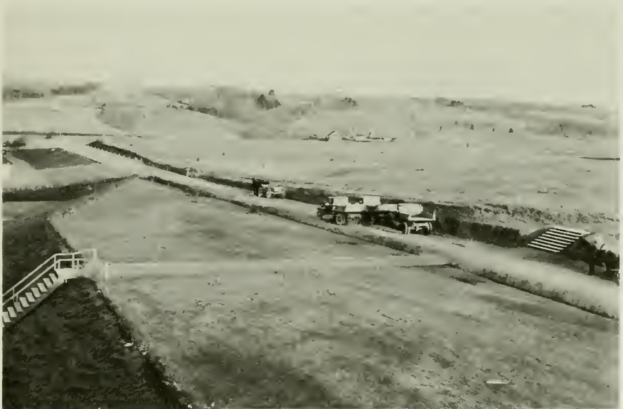
Work on the recreational field project (including the football field which became the new Mt. Olympus) began in December 1934. The project was completed by the Work Division of the State Emergency Relief Board.
