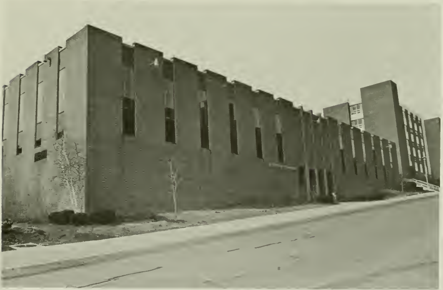
William W. Scranton Commons, on Second Street, southeast of Carver Hall.
