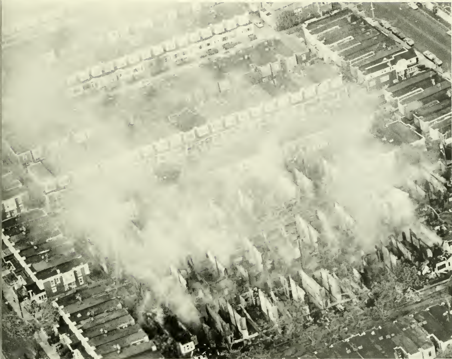
An entire city block was destroyed in May in Philadelphia. Police tried to evict members of the radical group MOVE from a fortified rowhouse by dropping a small bomb on the building. The device started a fire that destroyed 60 houses and 11 lives.
