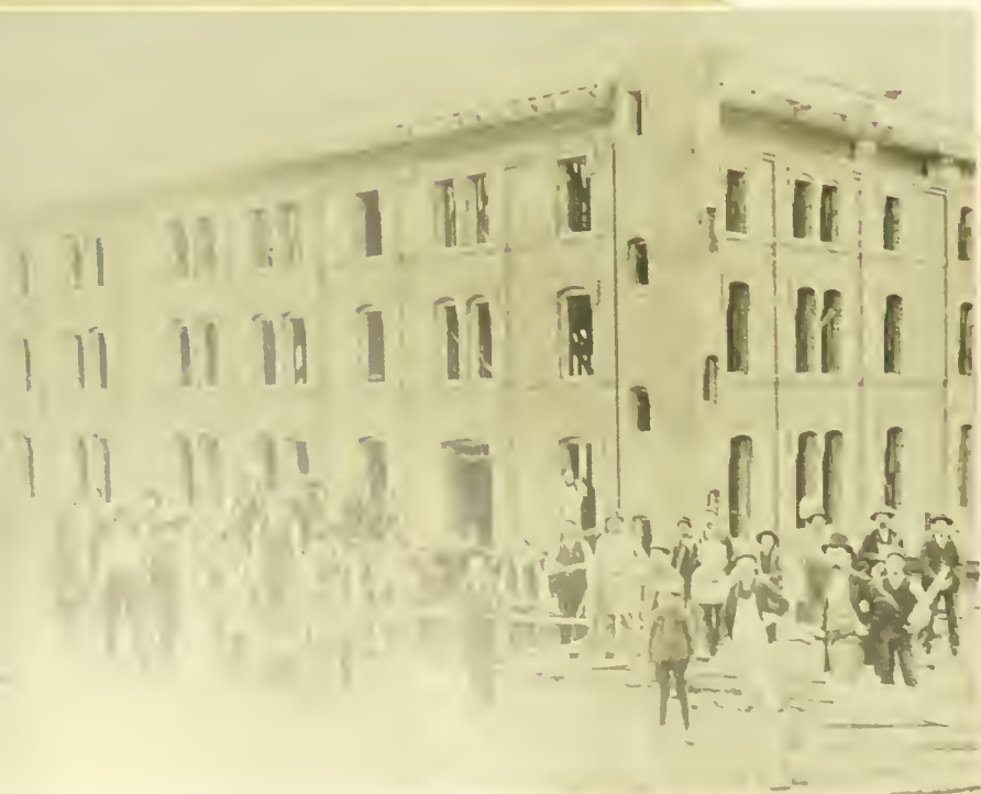
Featured here is Waller Hall undergoing construction in 1890.
