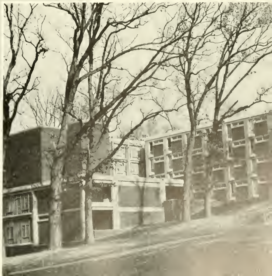
East Hall, shown here, and its counterpart, West Hall are the latest additions to the campus.
