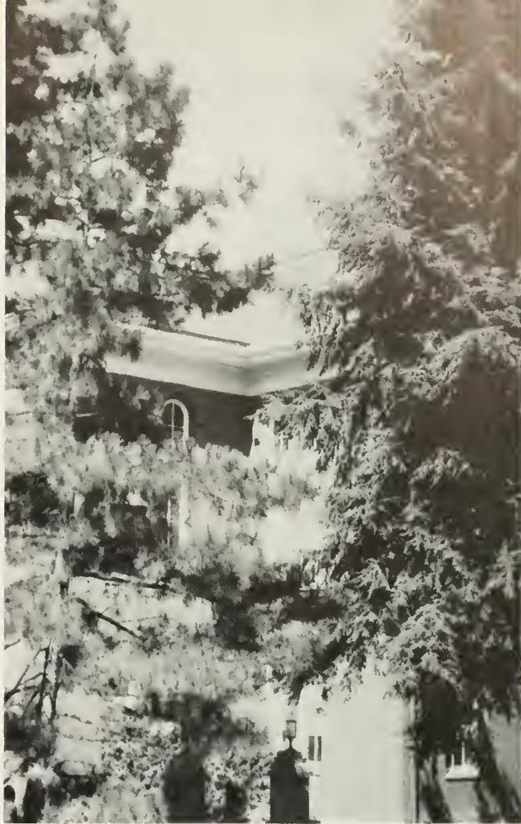
▲ Rear View of Carver Tower
