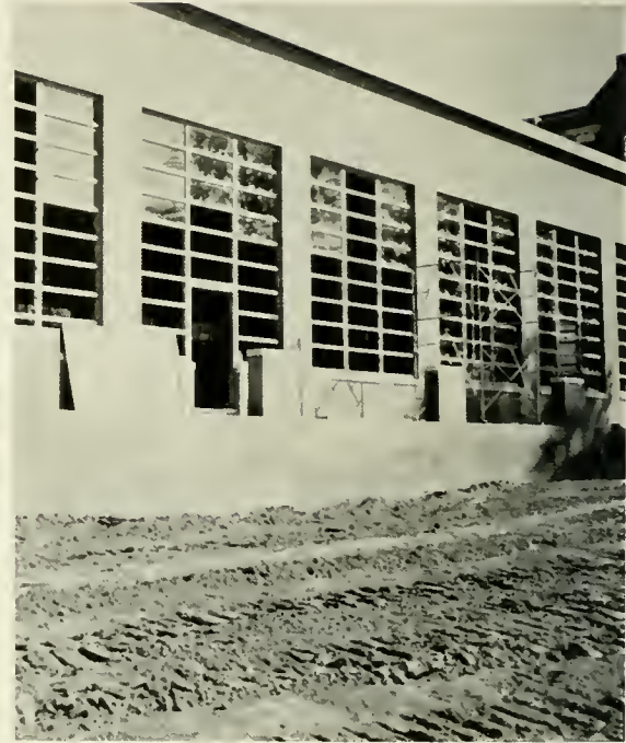
When the exterior was nearly completed.
