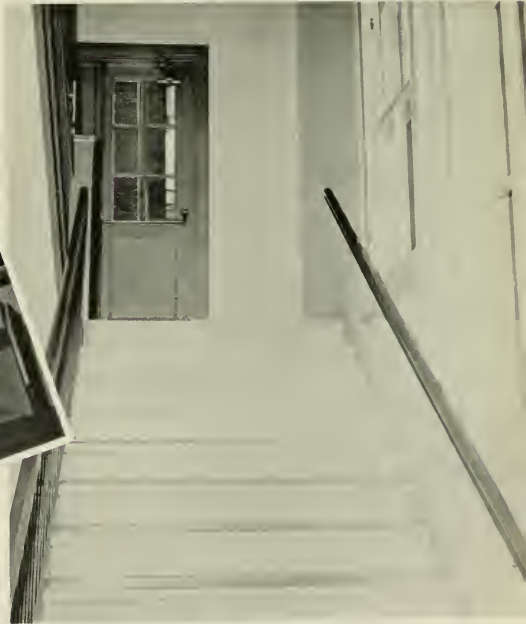
up the old familiar back stairs to . . .
