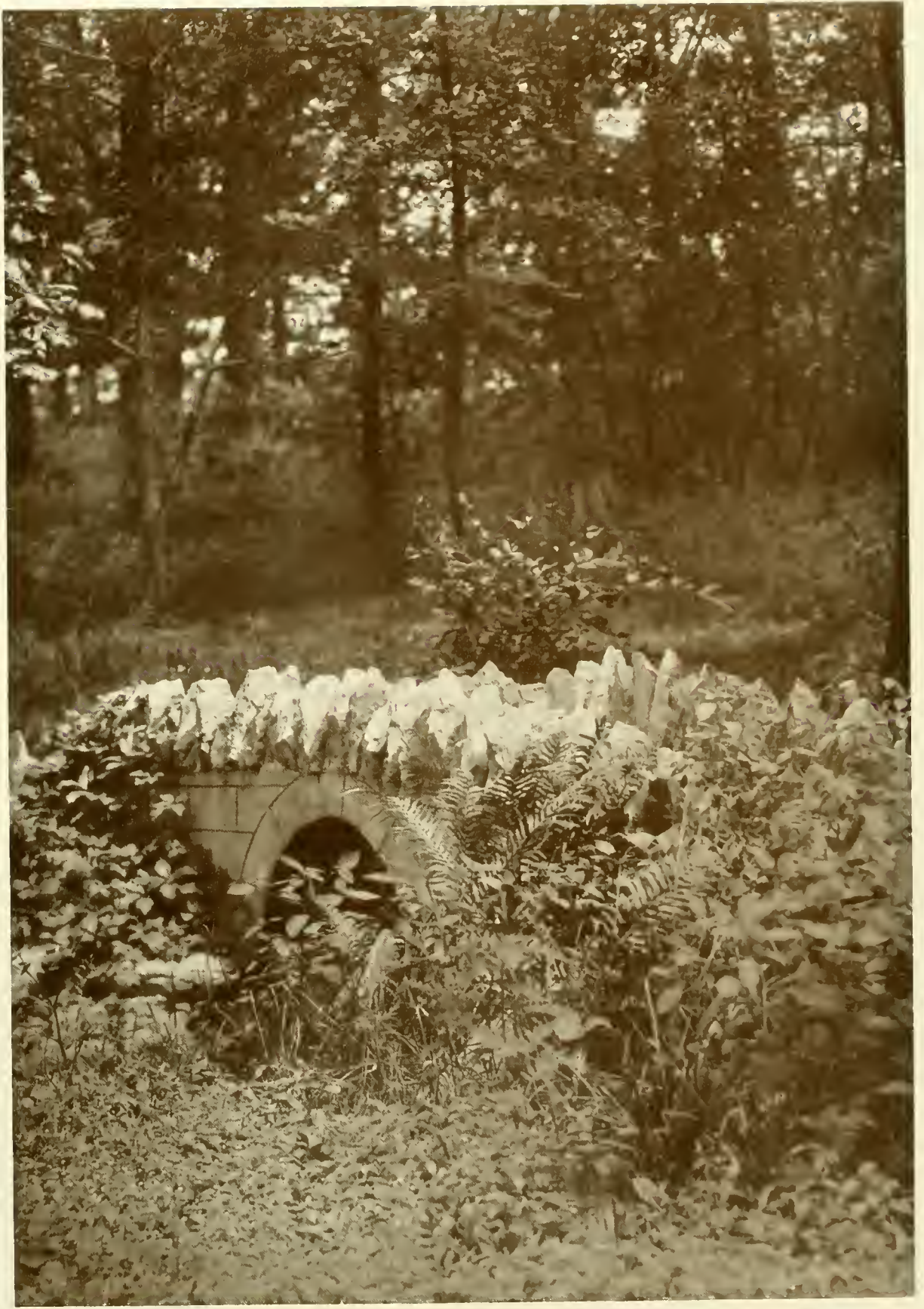
THE FOOT BRIDGE
