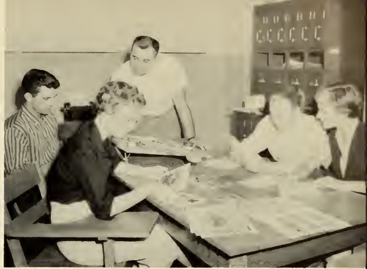
One of three student offices adjacent to Husky Lounge.
