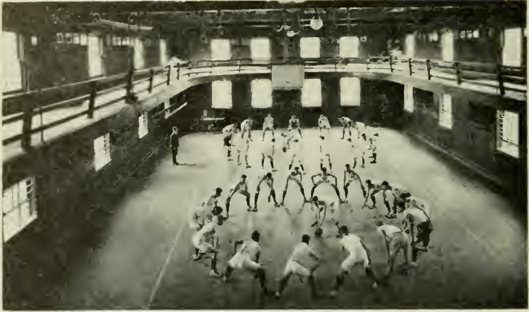
Old Gymnasium With Running Gallery—1921
