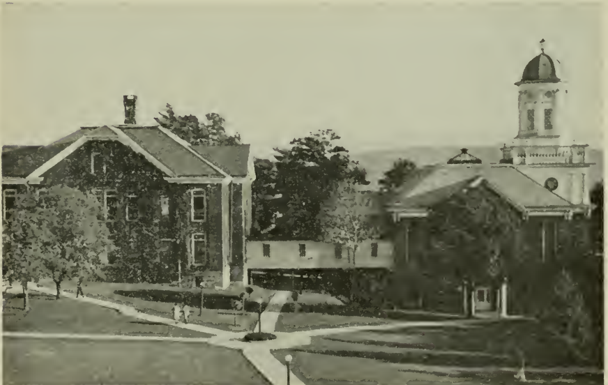
Bridge Connecting Noetling and Carver Halls—1939
