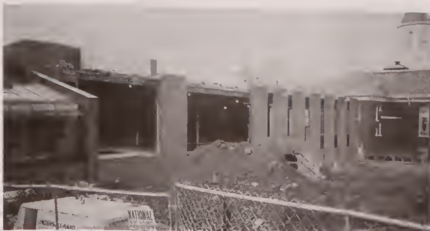
Extensive renovation of the Scranton Commons dining facility is underway.
