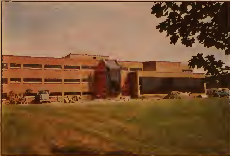
McCormick building nears completion
