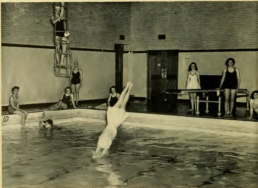
SWIMMING POOL CENTENNIAL GYMNASIUM
