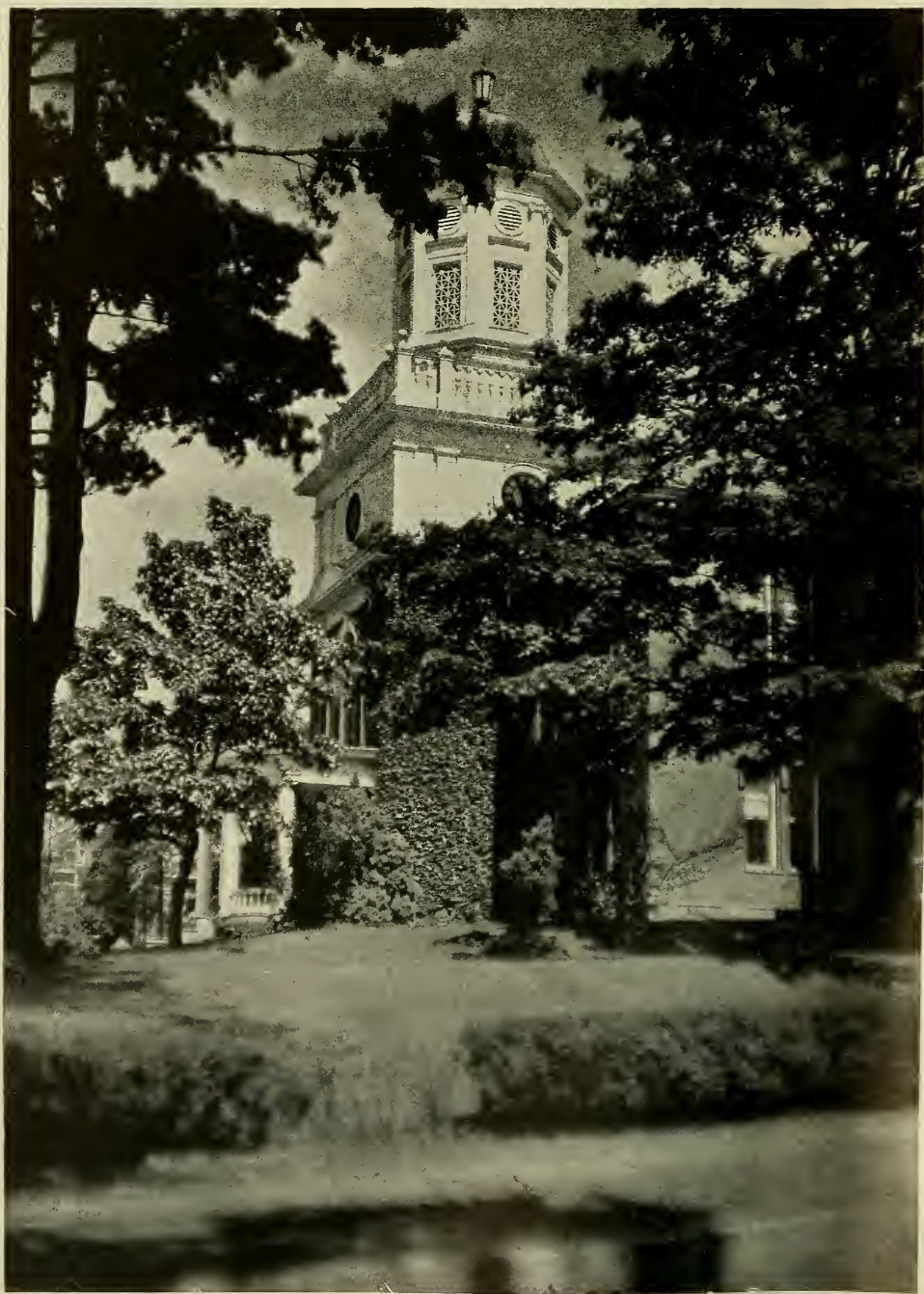
CARVER HALL ERECTED 1867
