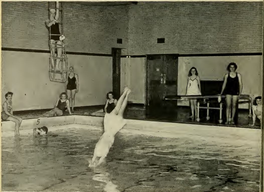
SWIMMING POOL CENTENNIAL GYMNASIUM
