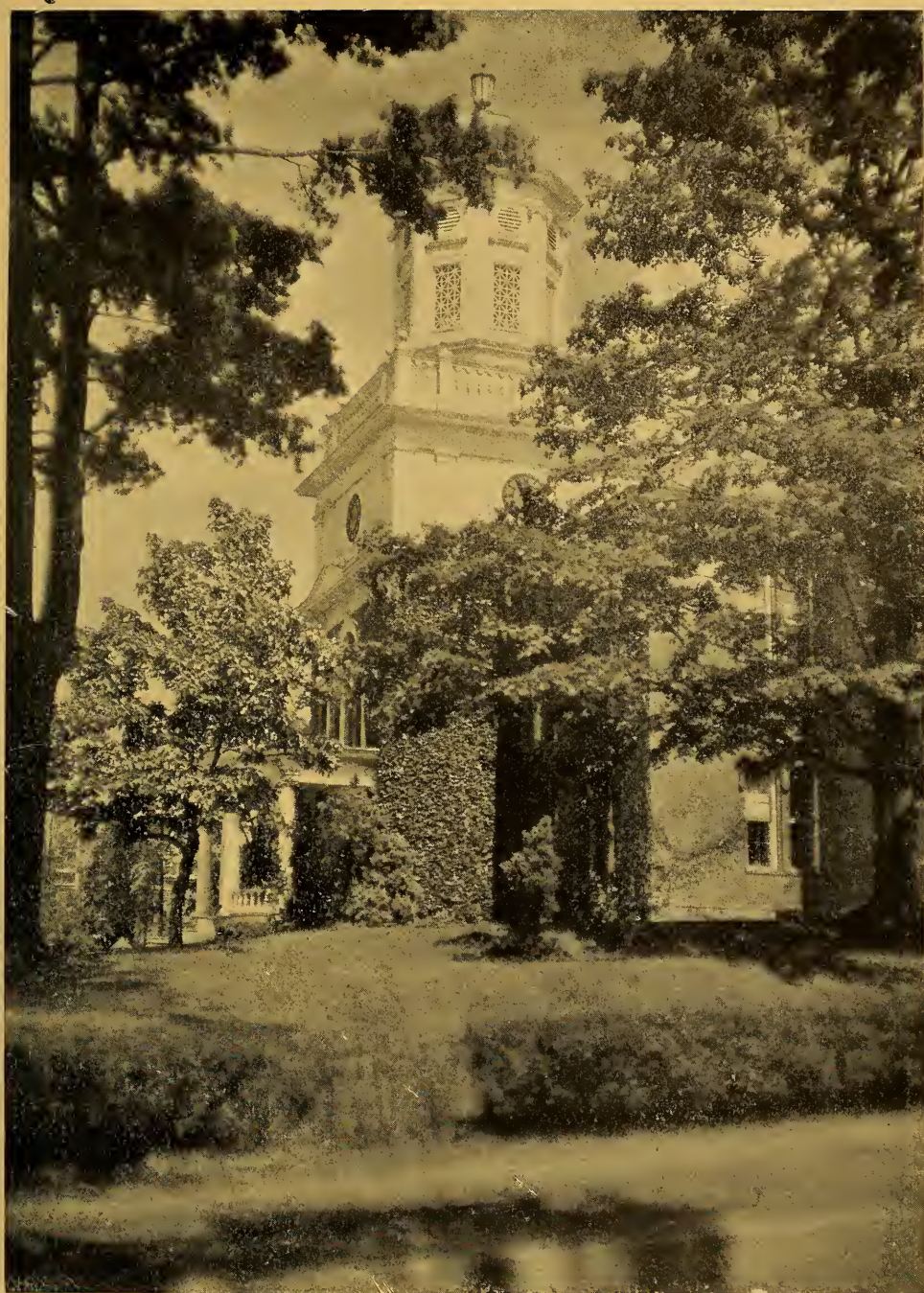
CARVER HALL ERECTED 1867
