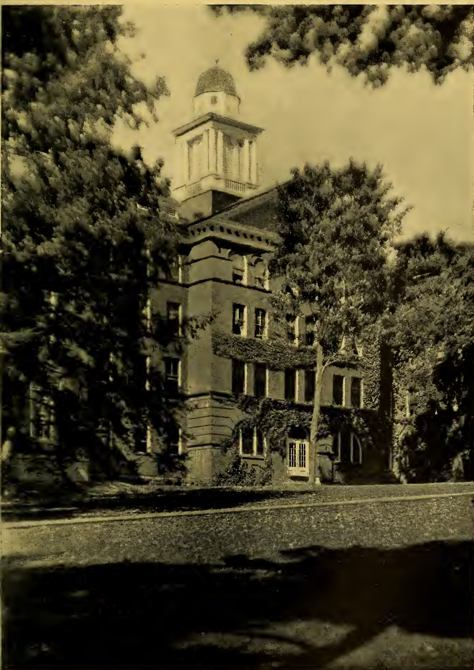
WALLER HALL—Containing Library and portion of Women's Dormitory
