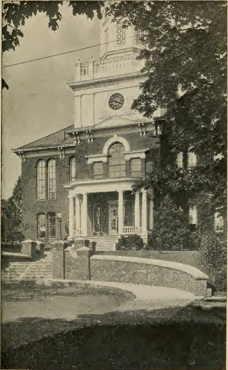
CARVER HALL, ERECTED 1867
