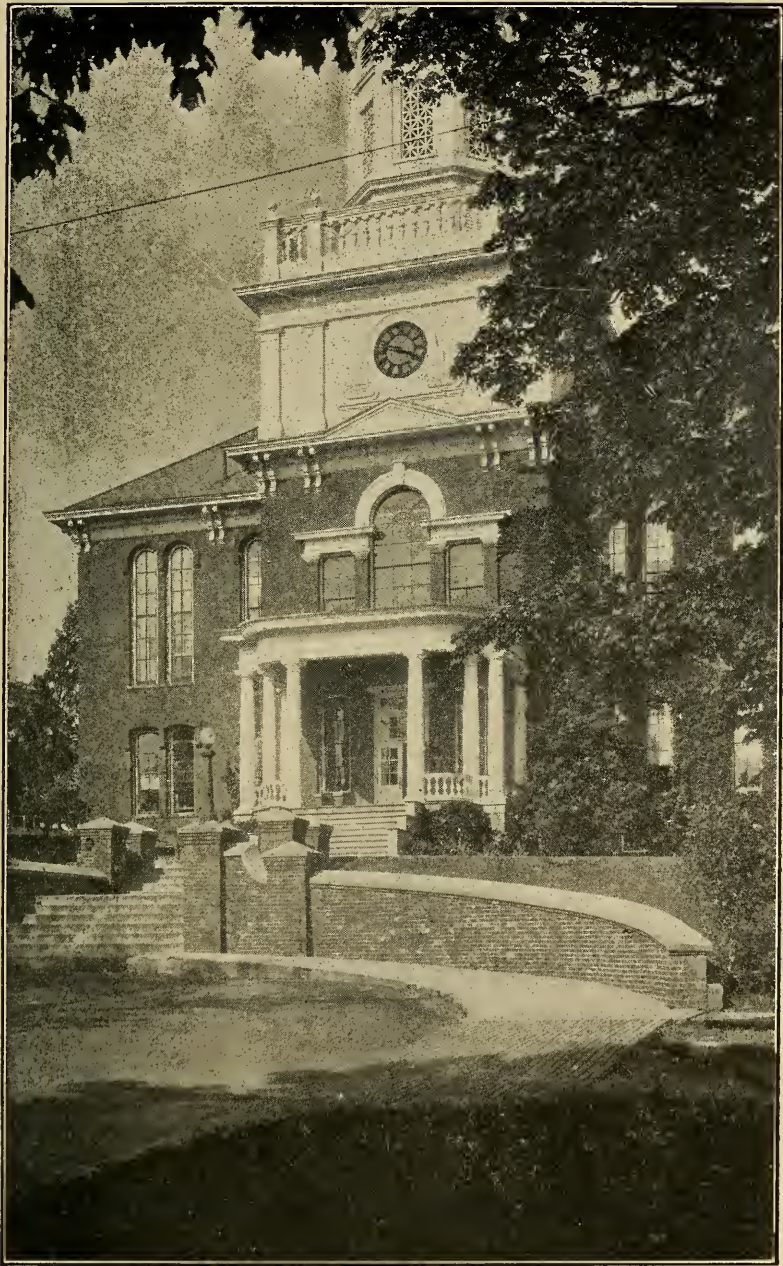
CARVER HALL, ERECTED 1867
