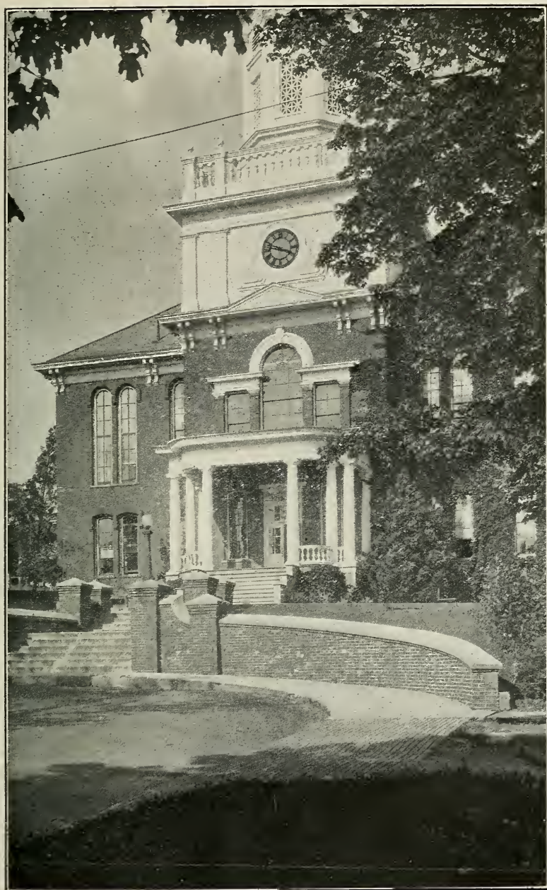
CARVER HALL, ERECTED IN 1867
