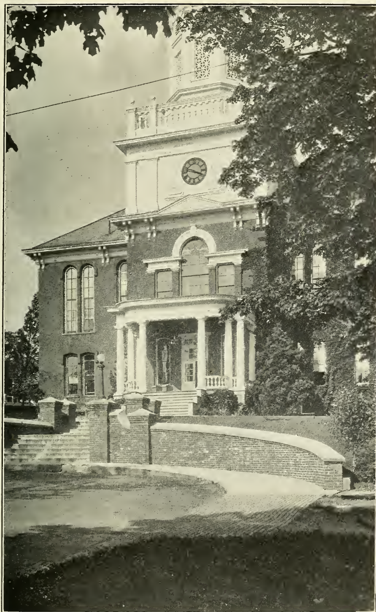
CARVER HALL, ERECTED IN 1867
